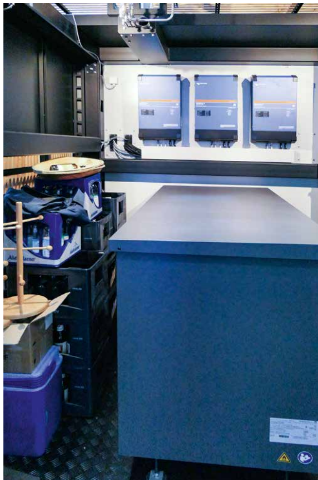
Fig. 2: Heat pump at the front and solar inverter on the wall [Photo: N. Petersen]
