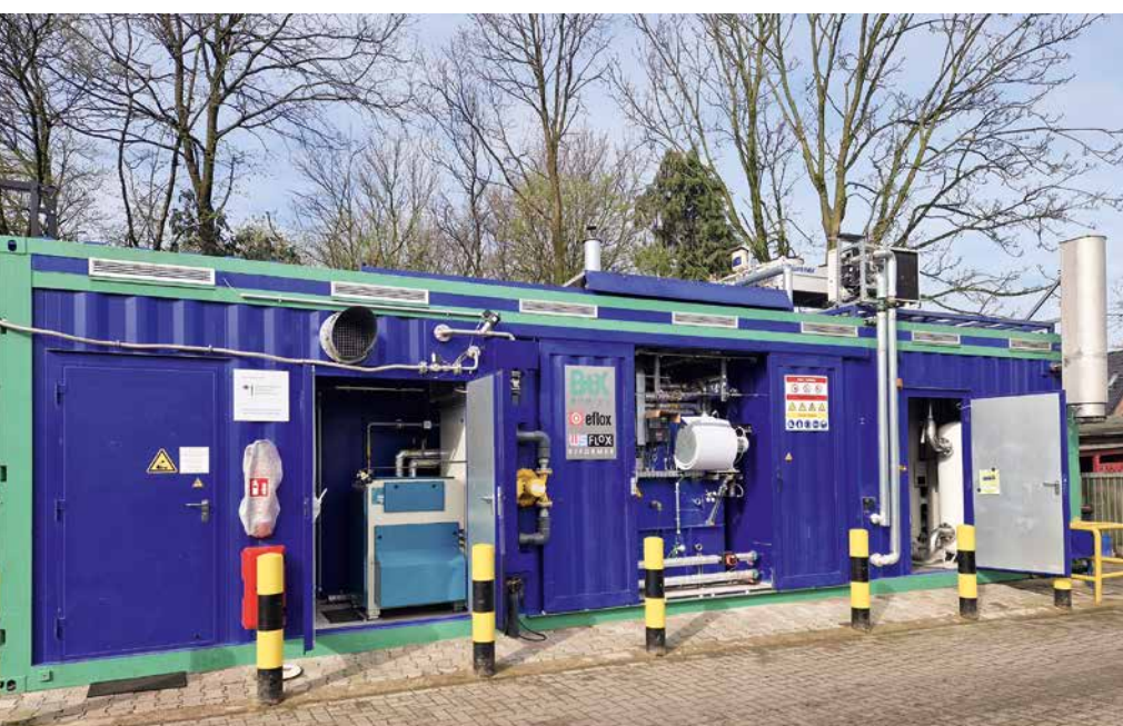
Fig. 1: Pilot plant for the steam reforming of biogas for the production of green hydrogen [Source: BtX energy]
